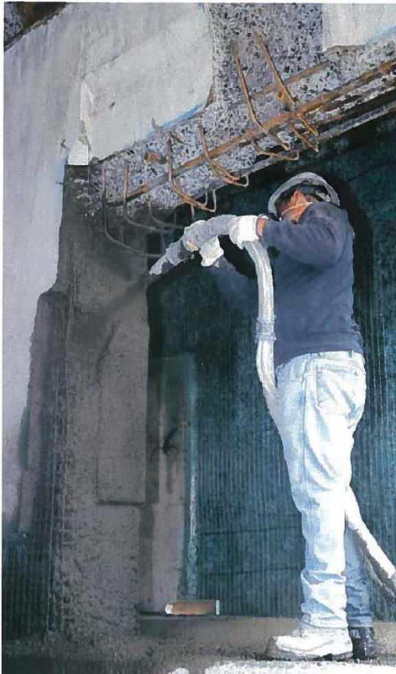
Fig. 2: City of Montreal - Overpass Shotcrete Repair
