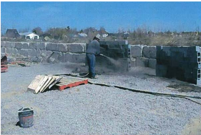
Fig.1: ACI Certified Shotcrete Nozzleman – Test Panel Shooting
