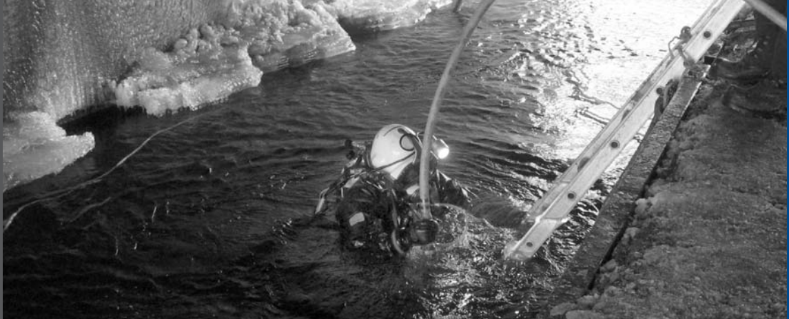
Photo credits : Simard-Beaudry Construction inc.
