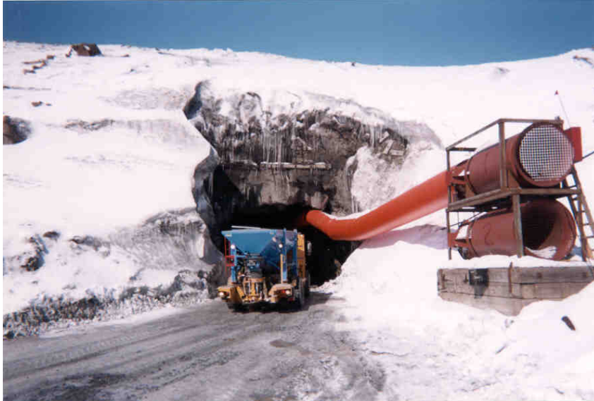
Figure 6: Shotcrete carrier using surface ramp access
