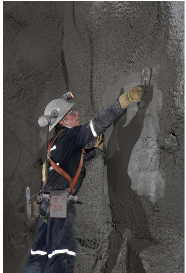
Trowelling of finish shotcrete layer
