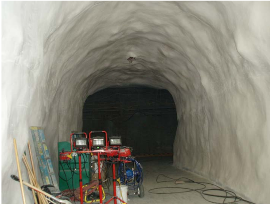
Painted walls of Ladder Room
