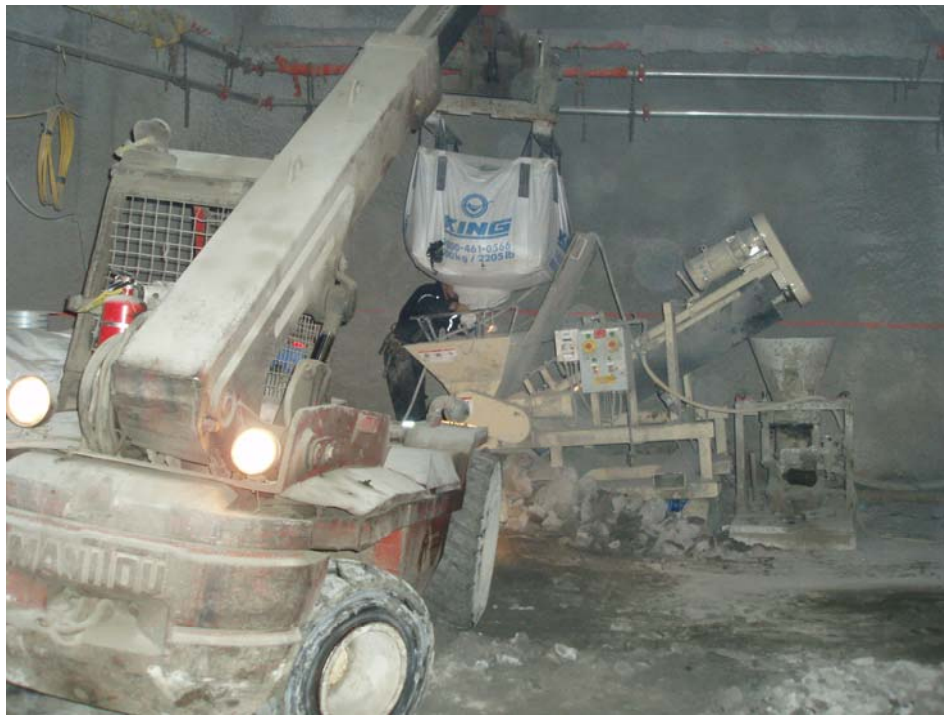
Shotcrete mixing and pumping equipment
