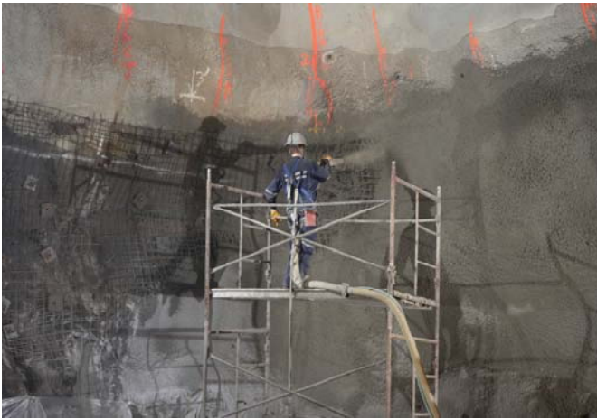
Shotcreting of drift walls in progress
