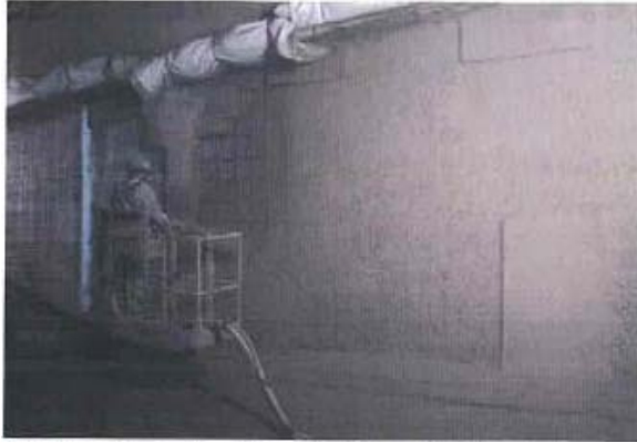
Fig. 9: Curing system already in place while
