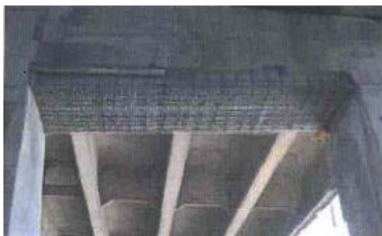
Fig. 6: Mesh installation- Île-aux-Tourtes Bridge
